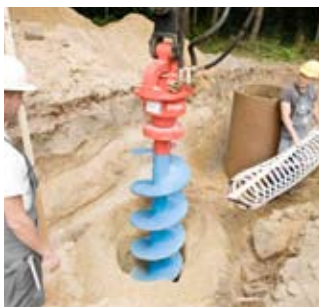
Typical auger drill bit used
